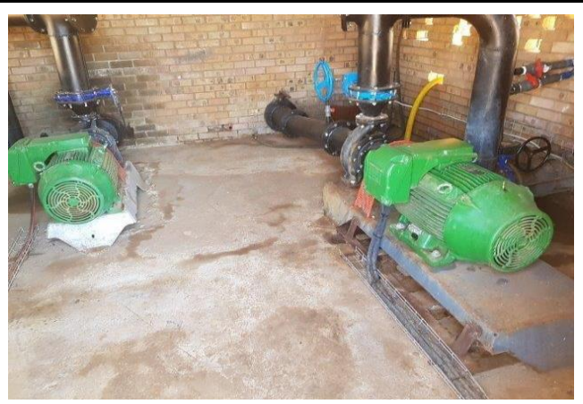
Pumps and infrastructure
