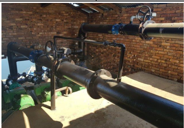
Pumps and infrastructure
