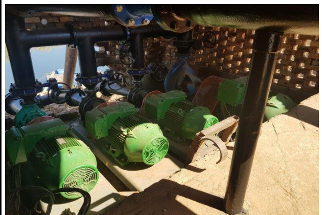
Pumps and infrastructure
