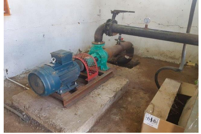
Pumps and infrastructure
