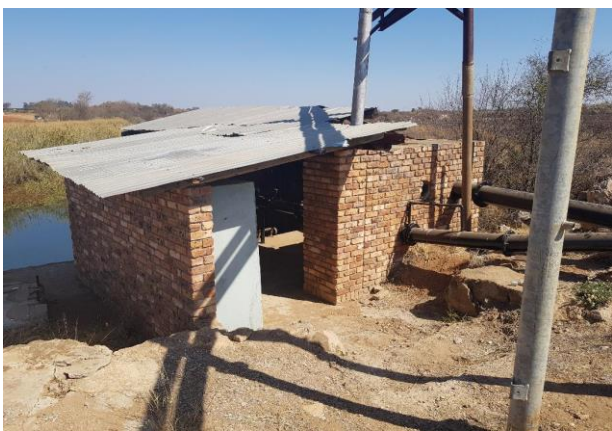
River Pump Station
